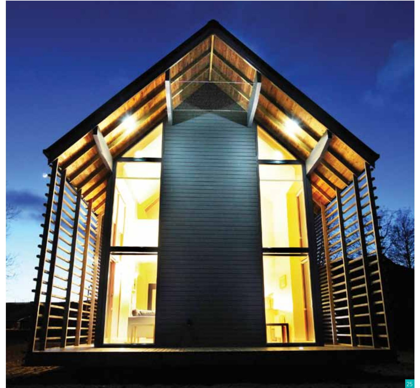
Model D House Architect: Gökay Deveci Client: Sylvan Stuart Ltd 'Passivhaus' standards Less than £900sqm Constructed from Scottish timber A sustainable, affordable and contemporary response to a rural Scottish vernacular – delivered by a design-led approach.
